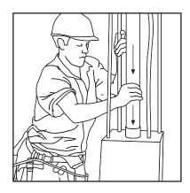
**2.-** 36 hours after pouring the column concrete, the Alsipercha can be used to: install boards, handrails, risers,...
