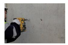
4.- Proceed to install the 4 chemical anchors per **Wall Bracket** (total 8 units of M16 stud bolts).
